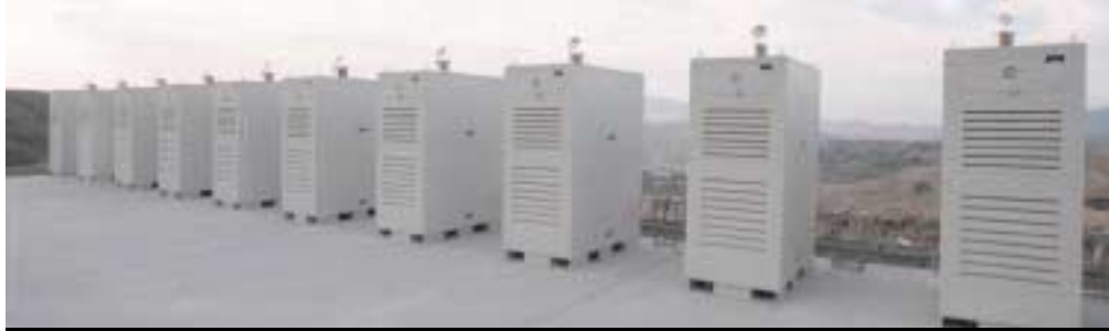
Figure 1. A ten unit array of microturbines running on biogas powers a Los Angeles landfill site
