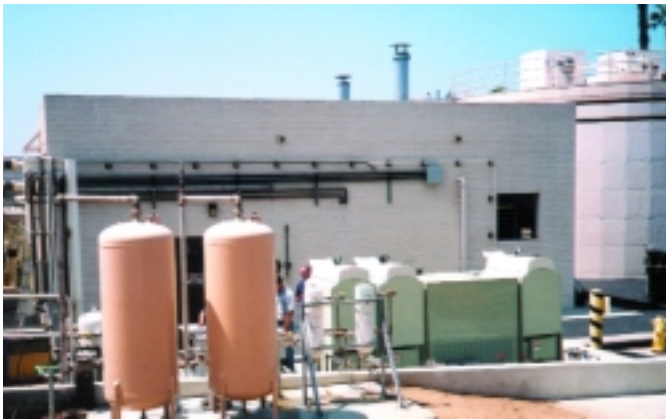
Two views of the microturbine installation at the San Elijo Water Reclamation Facility
